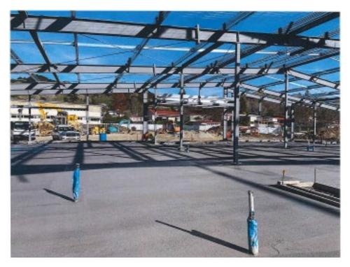
3.3 The carpark sub-base construction is well advanced with placement and shaping of basecourse to finish levels underway along with associated surface drainage (under review). Installation of steel framing to the gymnasium area is well underway and formwork to the perimeter of the amenities area is progressing. Pouring of the concrete amenities slab has been completed as has installation of the precast panels.
